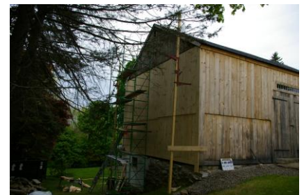
Barn after completion of north wall.
