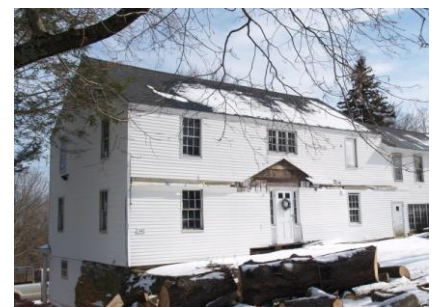
Barn as it appeared at the start of the restoration project.
